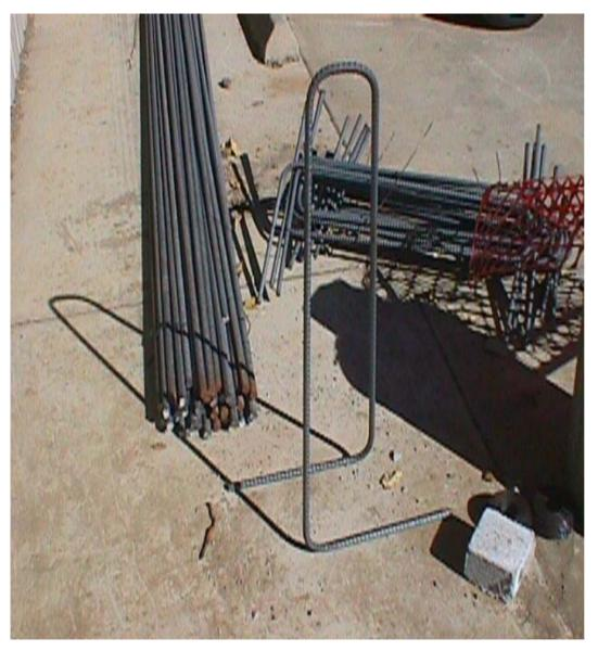
This is called a "standee". These typically come from your rebar supplier and are bent per your specs. They get tied to the lower grid to support the upper grid.
